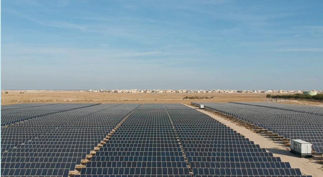
Figure 2. PV Solar Energy with RO has been implemented since 2016 in Khafji, Saudi Arabia. The KACST project has a capacity of 60,000 m 3 /day
